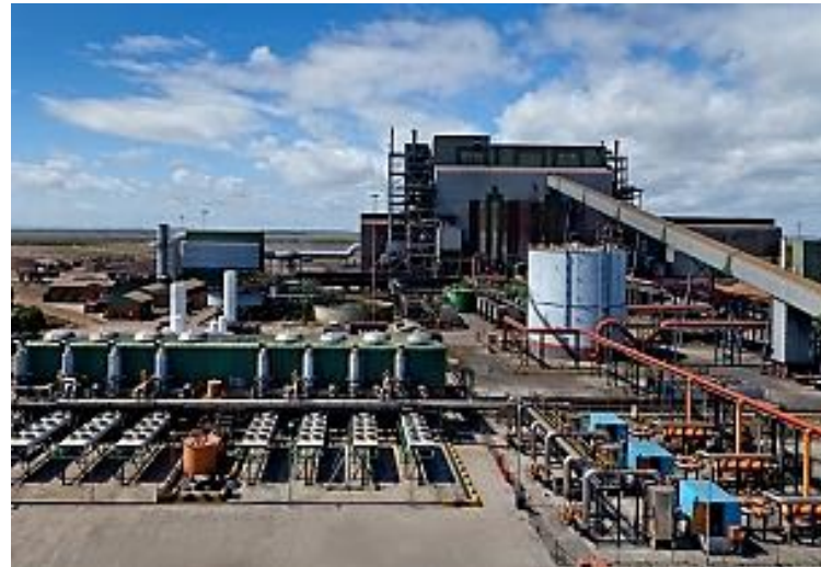
Prime Power Plant (Low Speed, Gas Powered)
